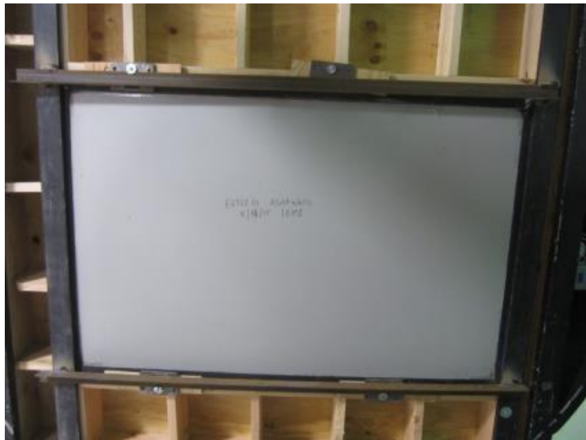
Photo No. 2 Post-Test Condition of Wall Specimen, Interior
